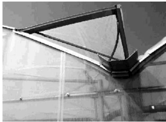
圖 2b. 屋簷式連續天窗 (Gutter-Wing)
