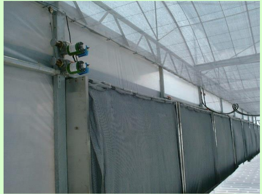
View from inside
